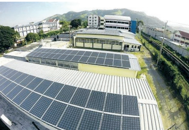
An aerial view of the section of the PV system located at UTech, Jamaica's Papine campus.
